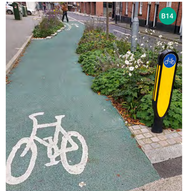
Picture B14 Rain gardens and cycleway in Altrincham, Greater Manchester.
